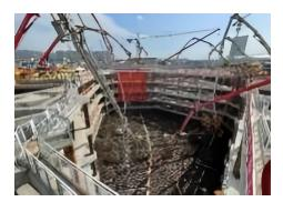
The microbial repair agent for concrete cracks was applied to the side walls, showing good effects on both crack repair and prevention. The average crack spacing was reduced to 1/2.5, the crack length was shortened to 1/2.8, and the number of cracks was reduced to 1/2.3. The ultrasonic wave speed after repair was greater than
