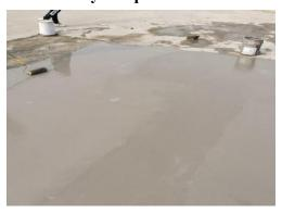
Due to severe surface deterioration of the road at a Nanjing factory , a rapid repair material based on sulfoaluminate and prepared with ART-P180 was used. This repair material meeted the self-leveling process requirements. It achieved a compressive strength of over 25 MPa within 4 hours and a bonding strength of 1.4 MPa, allowing for the quick restoration of traffic conditions. Furthermore, the compressive strength reached 48.5 MPa at 1 day.
