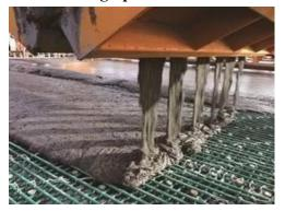
During the casting process of a UHPC (Ultra-High Performance Concrete) bridge deck panel, a pre-mixture was formed by using ART-P180 in combination with the cementitious material, and it was mixed and poured on-site. ART-P180 significantly reduced the viscosity of the UHPC mixture and enhanced its flowability and ability to release trapped air bubbles. The on-site production test blocks achieved a compressive strength of 147.6 MPa at 28 days.
