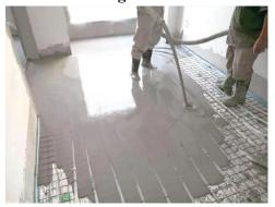
A construction company used C30 self-leveling floor mortar to achieve floor leveling in the interior of a residential building. The requirement was to achieve rapid hardening and reduce surface roughness. By using self-leveling floor mortar prepared with ART-P180, they achieved hardening within 4 hours, enabling walking capability within 6 hours. The self-leveling floor had a thickness of 4mm and a flatness within the range of 1-2mm/m.
